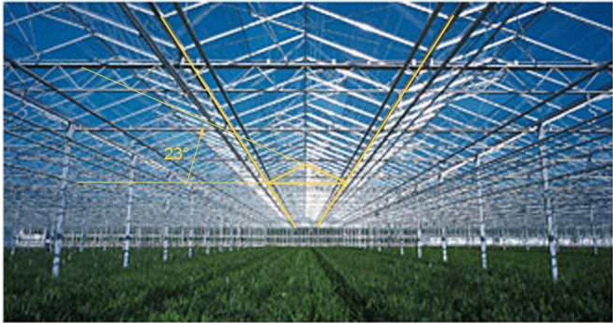
Fig.29. Typical “Venlo” style glasshouse on Guernsey with 2m x 1m glass panes laid to a ridge angle of ~23°. Other “Q22” glasshouses have 75cm panes inclined at ~30° and are built in multiples of a 7m span. (Photo courtesy Paul Ingrouille, Guernsey Clematis Nursery Ltd.)
